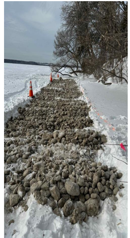
As illustrated, the strip of stones are installed 4.0m to 8.5m from shore.
